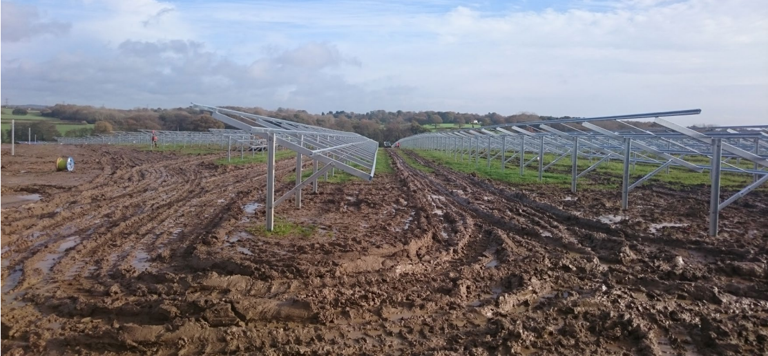
Inserts 36 and 37: Winter Installation (2015) and Operational Site (2022)
