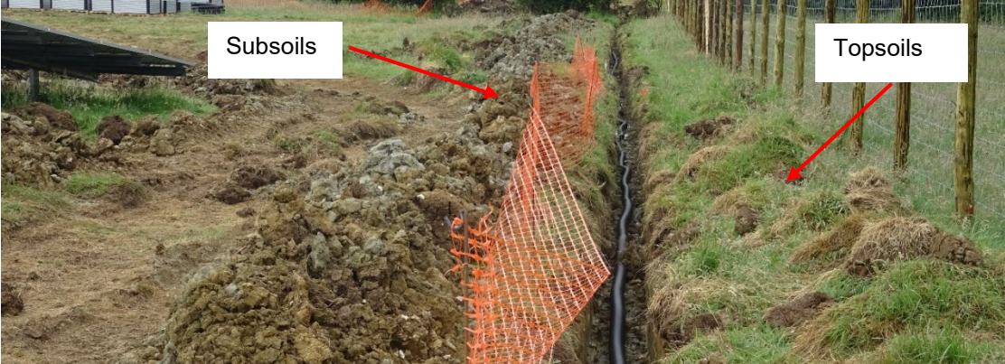
Insert 42: Subsoils Dug out of the Trench
