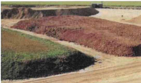
Clearly defined stockpiling of different soil materials
